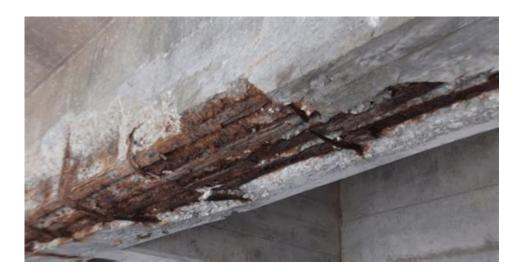
**Corrosion of steel in concrete** is a significant issue that affects the durability and longevity of reinforced concrete structures. Steel is commonly used in concrete to improve its tensile strength, but when the protective concrete cover is compromised, the steel can corrode, leading to structural failure. This article will explore the mechanisms of corrosion, the factors contributing to corrosion, its effects on concrete structures, and the methods to prevent and mitigate this problem.
