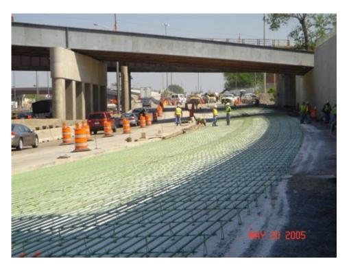
Continuously reinforced concrete pavement (CRCP) is an advanced pavement technology that has gained traction in the construction and maintenance of roadways. This innovative system employs continuous steel reinforcement embedded within concrete to create a durable and long-lasting surface. As urbanization and traffic volumes increase, the need for efficient and effective paving solutions becomes paramount, making CRCP a pivotal choice for modern infrastructure projects.
