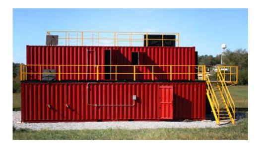
**Container fire training building** systems have become an essential component in the training arsenal for firefighters and emergency responders worldwide. These innovative structures provide a realistic and safe environment for conducting fire drills, allowing trainees to develop vital skills and experience. In this article, we will explore the features, benefits, design considerations, and types of container fire training buildings, as well as their significance in firefighting education.
